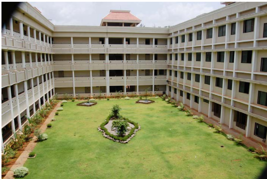
Inner View of Main Block
