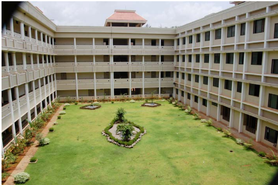
Inner View of Main Block
